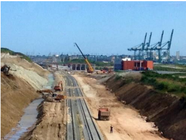
Building the railway to Mariel
